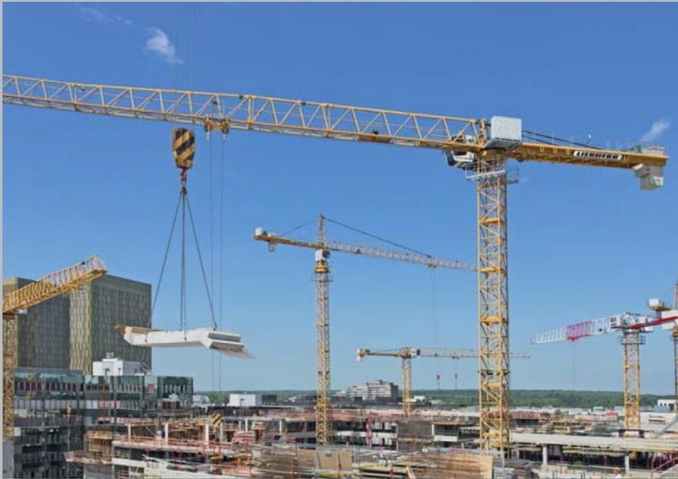
**Challenge:** Numerous joints need to be bolted together during the erection of a tower crane. The stability of the tower crane is dependent on the integrity of its bolted sections. The precise application of torque is critical to ensure the tower crane's stability.
